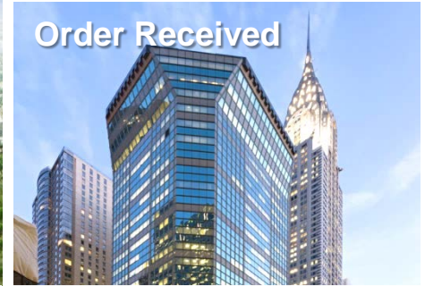
425 Lexington Avenue (New York, USA) Modernization for existing elevators: 14 units
