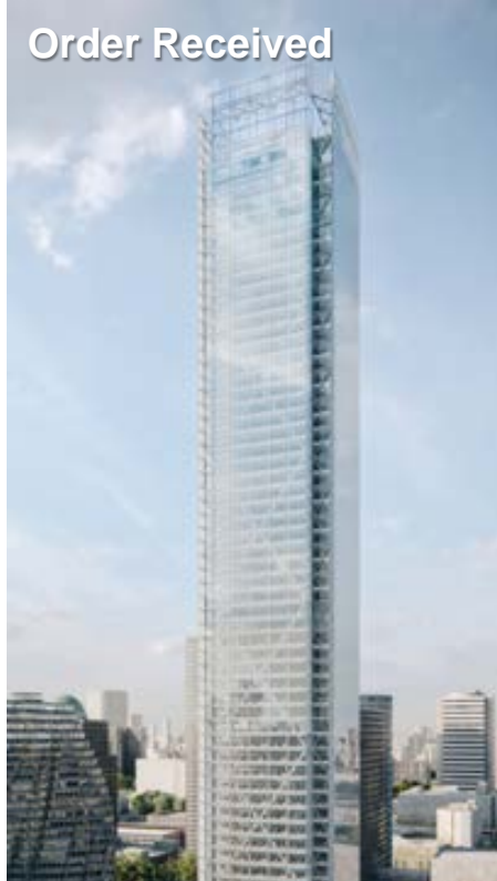
Fubon Xinyi A25 (Taipei, Taiwan) Elevators and Escalators: 33 units
