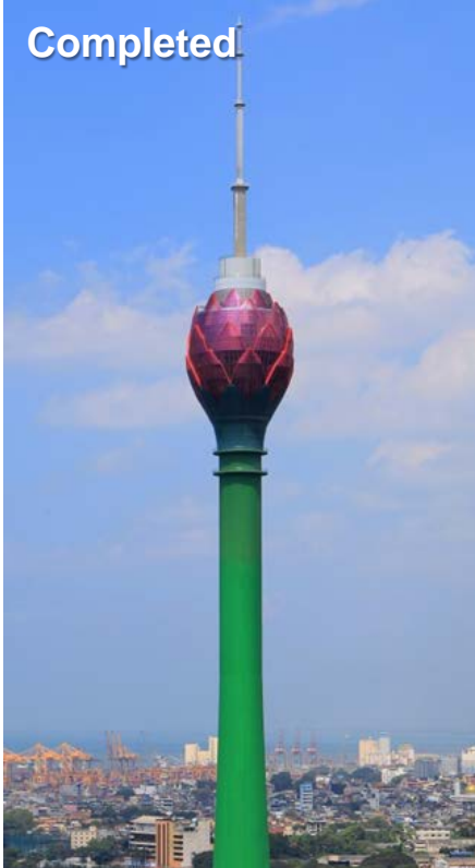
LOTUS TOWER (Colombo, Sri Lanka) Elevators and Escalators: 14 units
